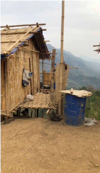
Bamboo shelter, Trade Center Camp, Lawngtlai District, Mizoram, India. Photo by CAM delegation.
